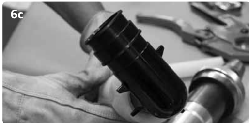
ProPEX Fitting Inserted into 2" Uponor PEX Piping
