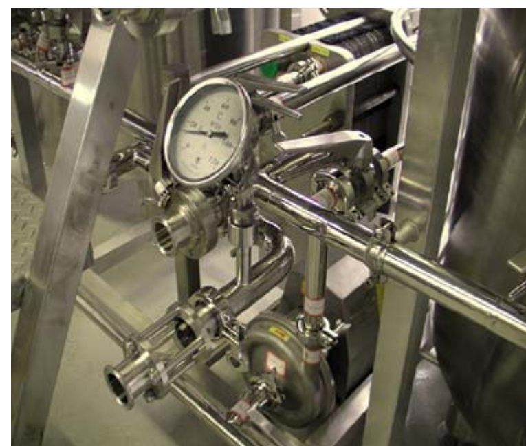
Wort out of the heat exchanger with thermometer and sight glass.
