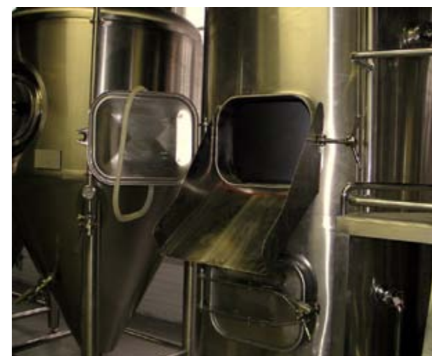
Grain out manway and grain chute installed.
