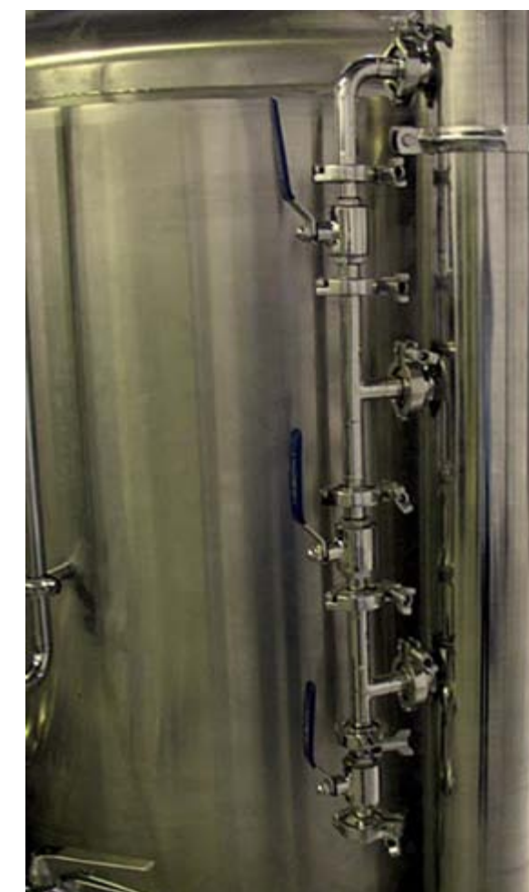
Condensate stack and water spray control.
