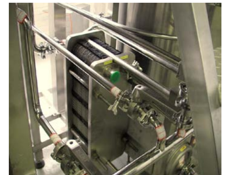
Heat exchanger and stainless steel hard piping set up.
