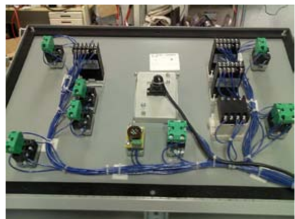
Control panel wiring.
